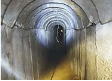
Sophisticated reinforcement of Hamas tunnel
